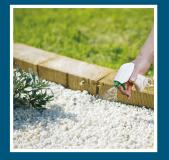
6. Apply the 3rd and final coat. 1 Litre covers 5m<sup>2</sup> in 1 coat, or the entire bottle would cover 15m<sup>2</sup>.
