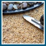
4. Straight after the second coat has been applied, compact or trowel the stones into place.
