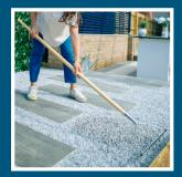
2. After the first coat has been applied, rake and agitate the stones to expose the uncoated stones.
