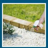
1. 1 Litre covers 5m<sup>2</sup> in 1 coat and 3 coats are required for a full bond. Ensure the depth of the stone is 20mm.
